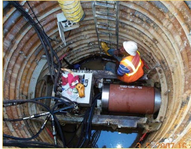
Workers were able to install 36 lengths of 1-m clay pipe — or a total of 118 ft in seven hours.
